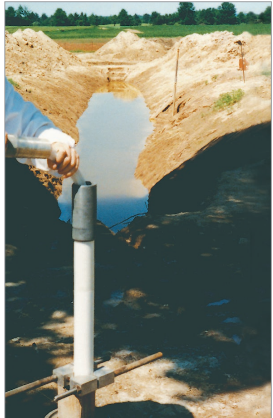
Underground oil pipeline leak assessment. Three 45 m (150 ft) installations. Two point rising head permeability tests were conducted in each interval of the Multilevel System. (See diagram showing contaminant distribution at left.)
