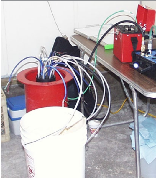
Four Waterloo Systems were installed to monitor a chlorinated compound release. Systems were installed at depths ranging from 430 ft - 750 ft, with most monitoring 7 zones. The Ports were constructed with both Double Valve Pumps and Vibrating Wire Transducers.
